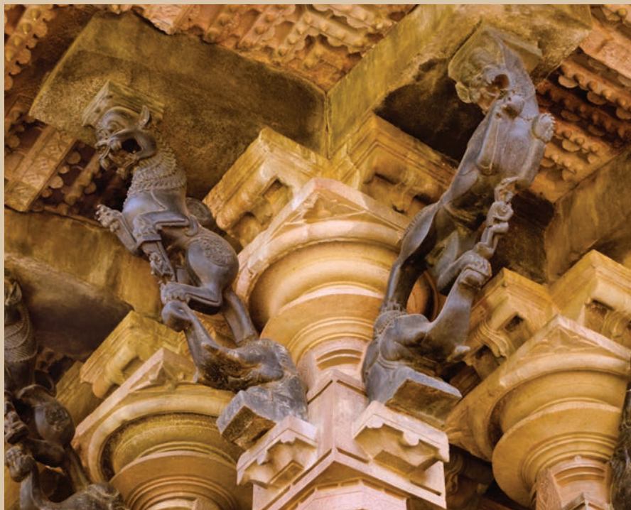
(L) Ornate pillar brackets made of granite were used to support the temple structure. (R) The sculptures of dancers and musicians carved out on the pierced screens
